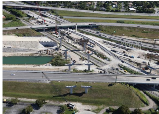
SW 120 TH STREET AT 122 ND AVENUE – LOOKING EAST
