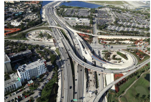
SR 836 WESTBOUND AT NW 42ND
