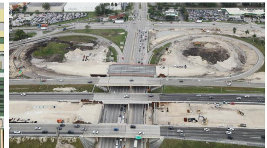
SR 836 AT 87 TH AVENUE – LOOKING EAST
